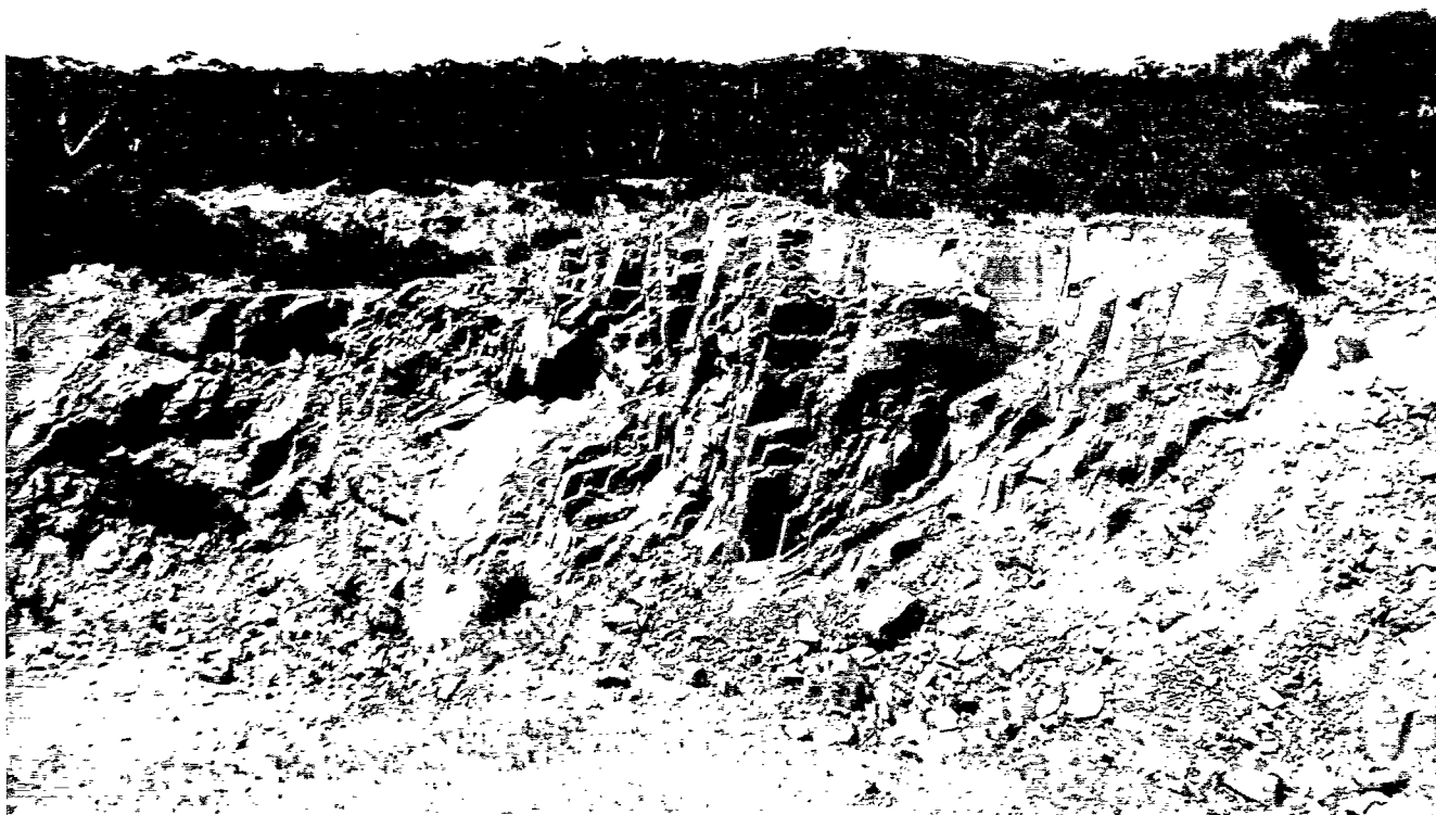
Southerly view of Mount Monster Quarry with the smaller quarry and conservation park in the background. Light coloured overburden of weathered kaolinitic porphyry in the face has a maximum thickness of 5 m (March 1981). Negative 34332.
